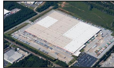
Newnan Distribution Center
