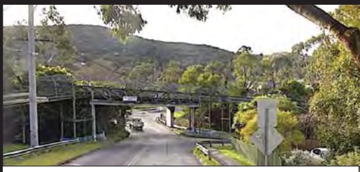
First shared-use trail was about 5 miles long with an overpass for bike path partially along railroad track
