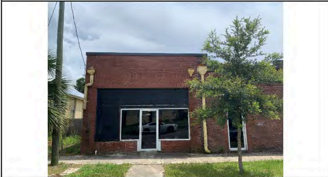
Photo 4: Partial northern elevation.
