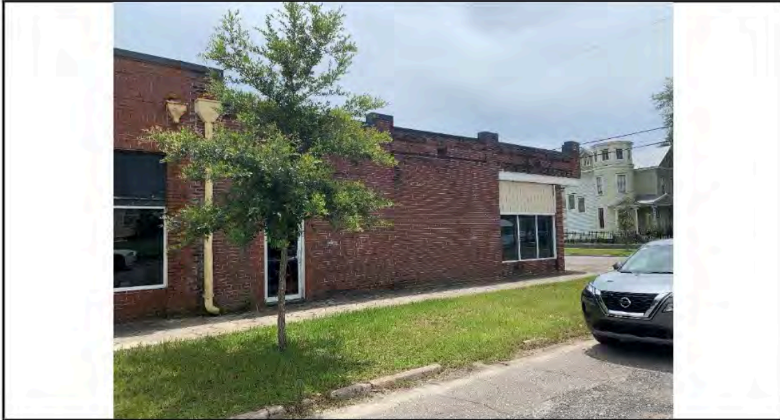
Photo 5: Partial northern elevation.
