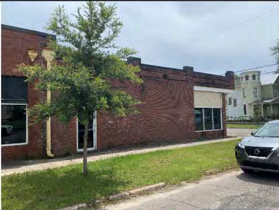
Photo 5: Partial northern elevation.
