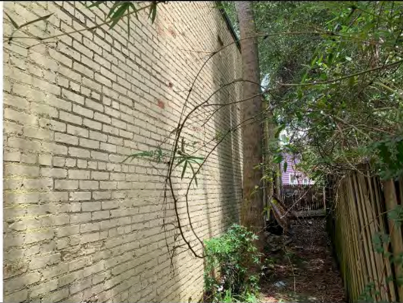
Photo 2: Partial southern elevation with wood fence to the right.
