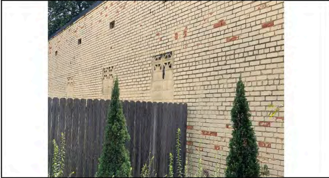
Photo 3: Partial eastern elevation – similar across entire elevation. Located along property line possibly.
