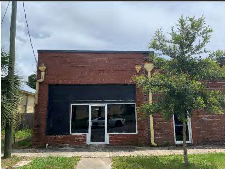
Photo 4: Partial northern elevation.
