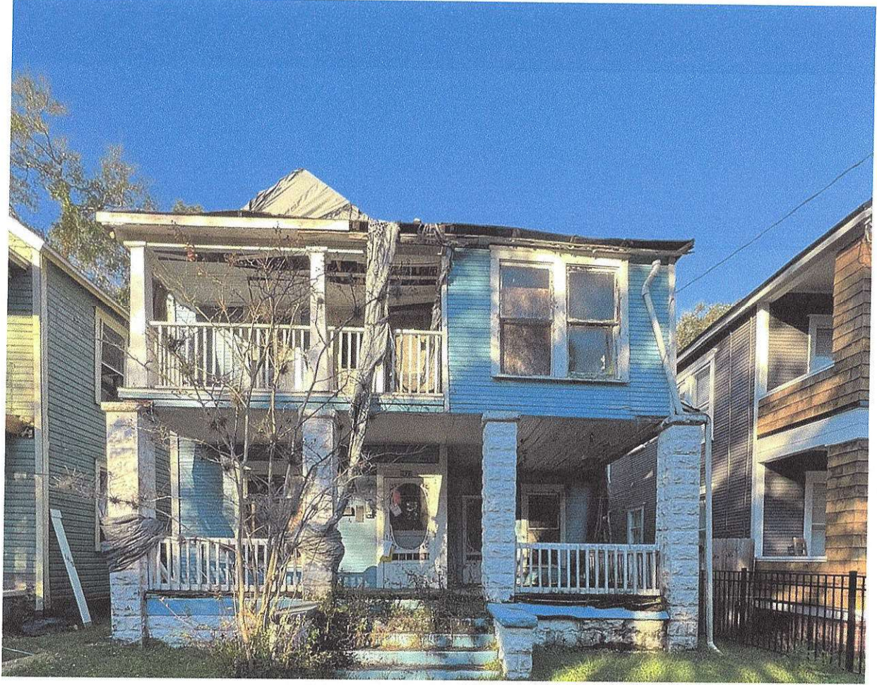
Photograph 1 The subject building
