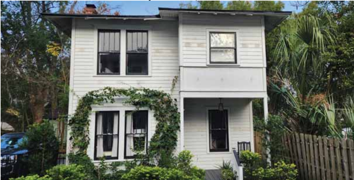
Accessory Structure (Built 1924)
