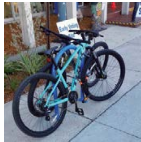
The Murray Hill Branch Library's inverted U-shaped rack provides bikes with support in two places, which is a crucial design component.
