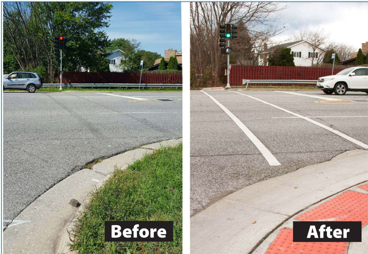
Figure 17. Photograph. A before and after photo of an RTA Access to Transit project that included the addition of a crosswalk, walk signal, and curb cuts to improve access to a stop on PACE's Harlem Ave. route in Palos Heights, IL (RTA, 2021).
