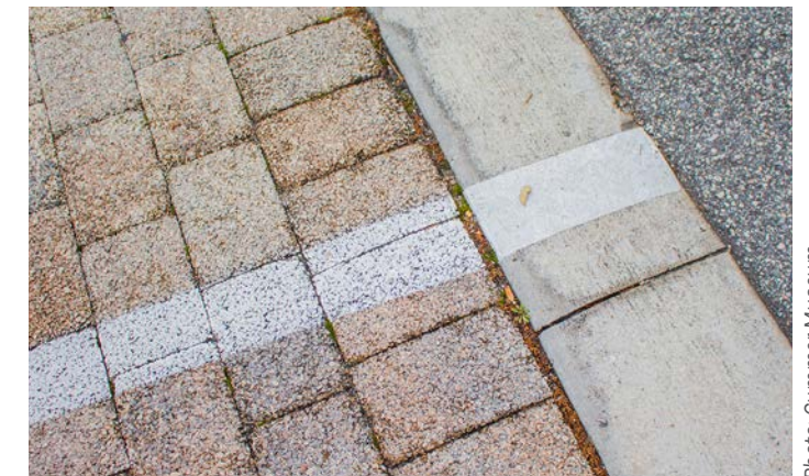
Permeable pavers in the Cummer Museum's parking lot allow water to infiltrate to the soil and reduce runoff while watering tree roots.
