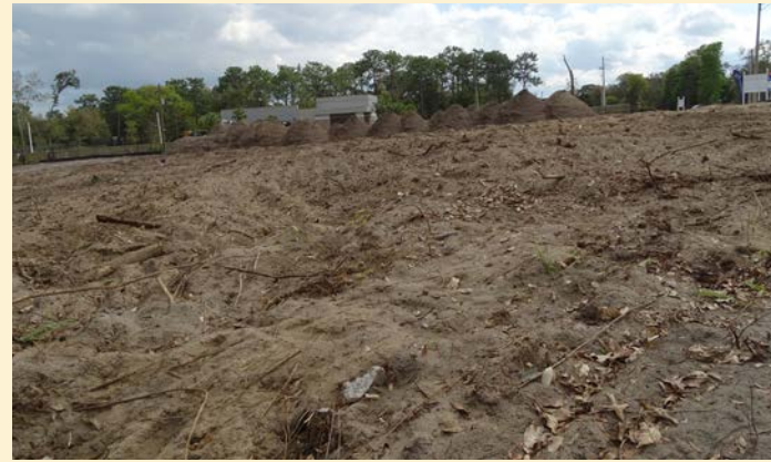
Total loss of tree canopy on a site that has been clear cut results in excess runoff and additional nutrient loading.
