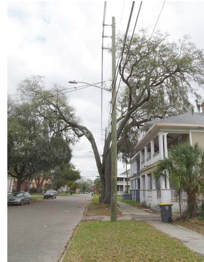
Too large a tree was planted under a powerline.
