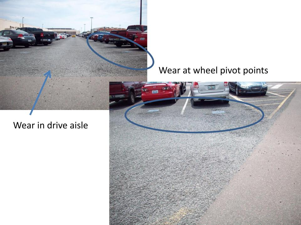
Solution: thin standard asphalt drive aisle and auto pivot points, Permeable detention space remains even under the asphalt: No changes to stormwater permit
