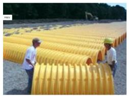
Figure 7 Installation of corrugated arch system, Figures courtesy of the following companies: ACF Environmental, Contech, GeoStorage, NTS, Raintank. Image 10 of 17
