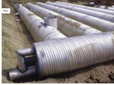
Figure 5 Cornugated metal pipe (CMP). Figures courtesy of the followin companies: ACF Environmental, Contech, GeoStorage, NTS, Raintank.
