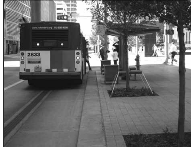
Figure 9.28 This bus stop is designed so that stormwater drains away from the curb into a slot drain located in the travel lane. This design keeps buses from splashing waiting passengers when pulling to the curb. Source: Texas Transportation Institute.
