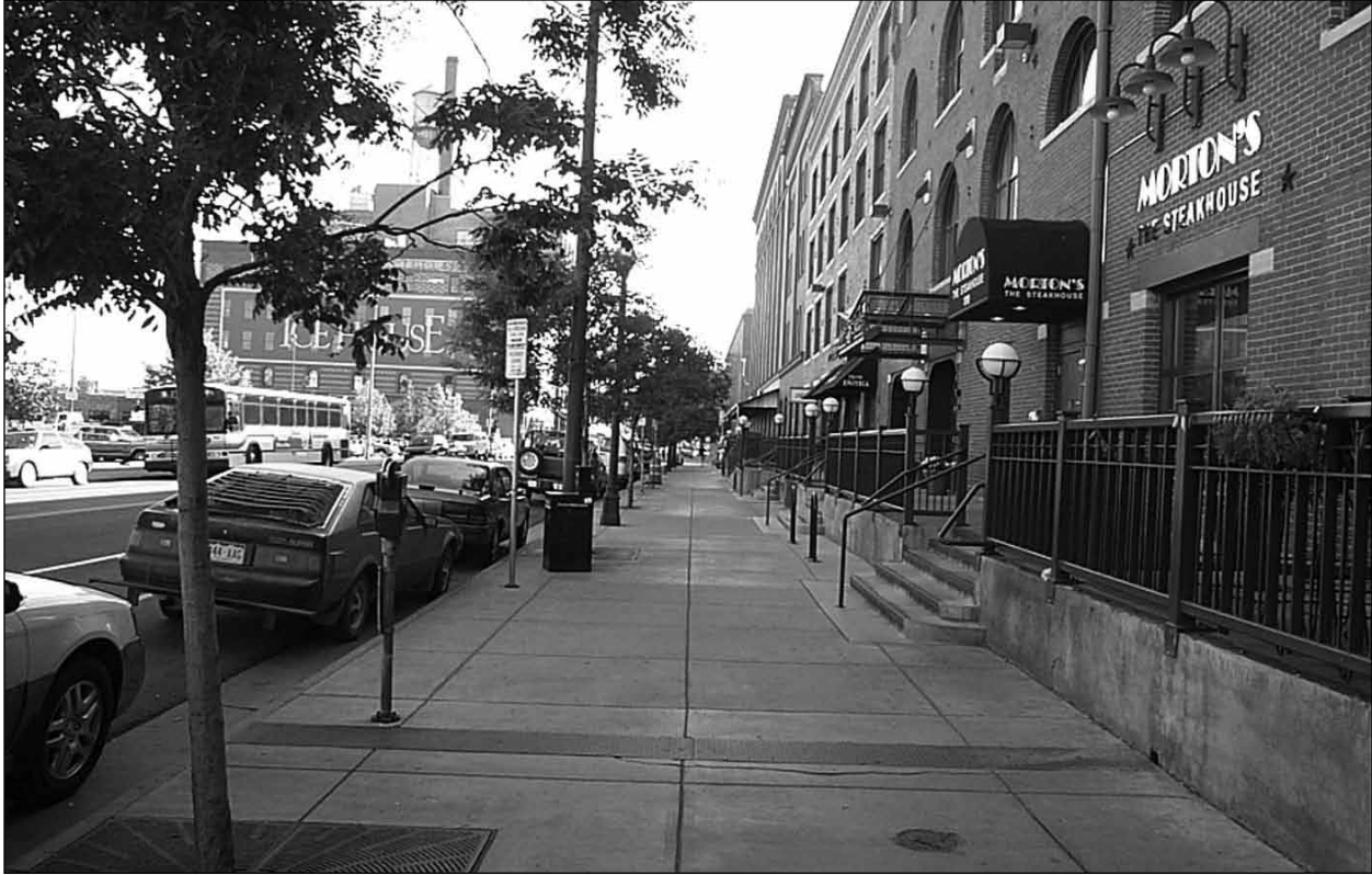
Figure 8.8 A combination of on-street parking, furnishings zone and wide pedestrian throughway provides ample buffer from moving traffic. Source: Kimley-Horn and Associates, Inc.
