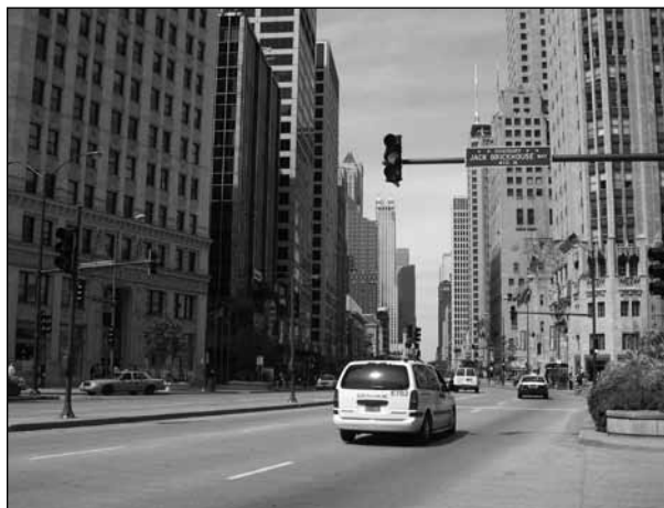
Figure 9.5 Narrow medians, such as on this boulevard in Chicago, should only be used to restrict turning movements, separate opposing traffic and create space for traffic control devices. Source: The Congress for the New Urbanism.
