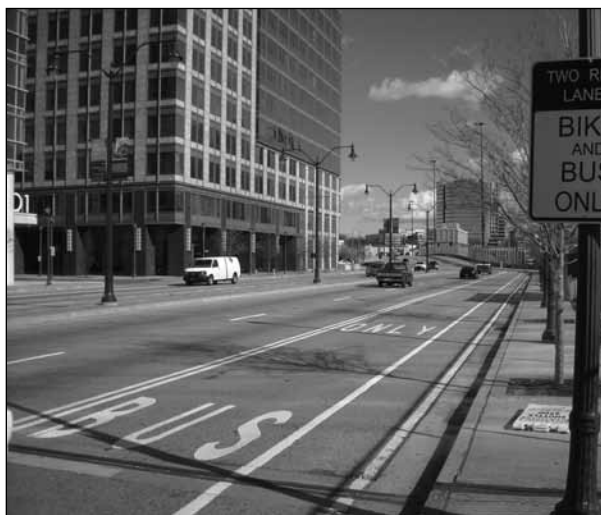
Figure 9.21 An example of a dedicated transitway in the outside lane of an urban thoroughfare. Note the bike lane located between the curb and the transitway. Source: Kimley-Horn and Associates, Inc.
