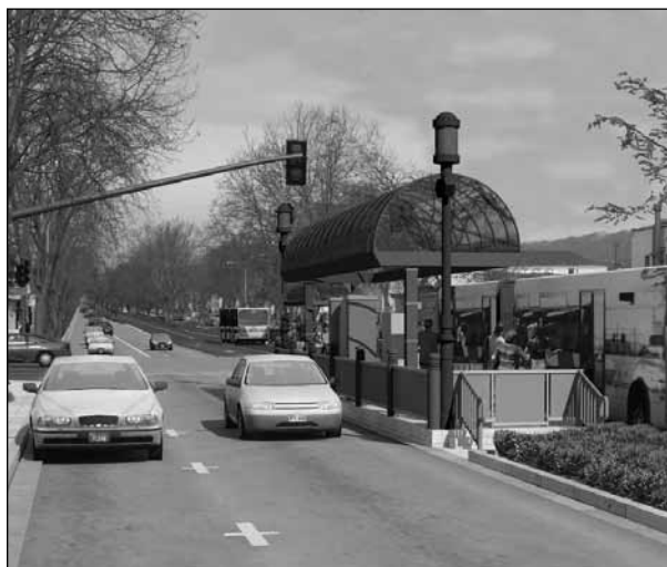
Figure 9.22 A simulation of a bus rapid transit center median station with dual outside platforms located at the far side of an intersection. Source: AC Transit.
