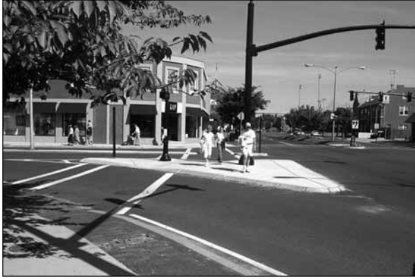
Figure 10.10 A channelized right-turn lane typically provides a pedestrian refuge island and an uncontrolled crosswalk. Source: Dan Burden, walklive.org.
