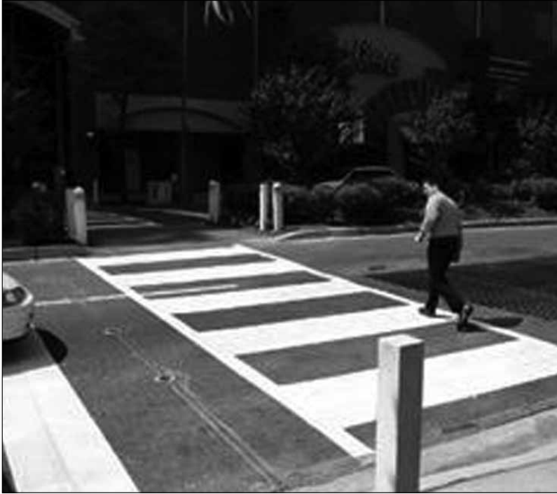
Figure 9.18 Midblock crossing with pedestrian detection and in-pavement lights. Source: Kimley-Horn and Associates, Inc.
