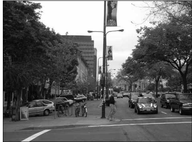
Figure 6.7 This multiway boulevard merges the access lane into the central roadway in advance of intersections. Source: Kimley-Horn and Associates, Inc.
