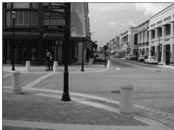
Figure 10.18 Use of contrasting material and bollards to delineate the pedestrian and vehicle areas. Source: Kimley-Horn and Associates, Inc.
