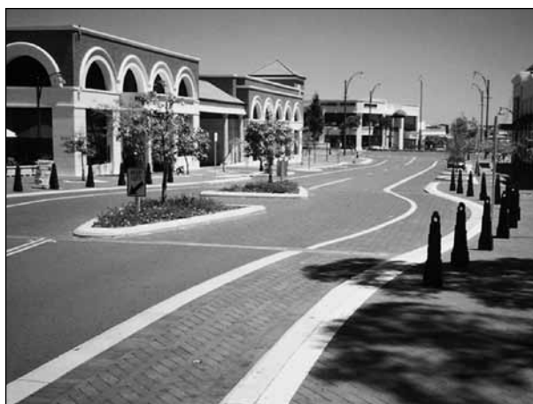
Figure 10.17 A mid block crossing with a flush curb in New Zealand. Pedestrians are separated from passing vehicles with bollards. Source: Community, Design + Architecture.
