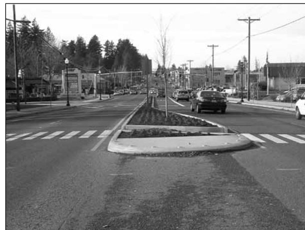
Figure 9.6 Median nose extended beyond the crosswalk to provide an enclosed pedestrian refuge. Source: Kimley-Horn and Associates, Inc.
