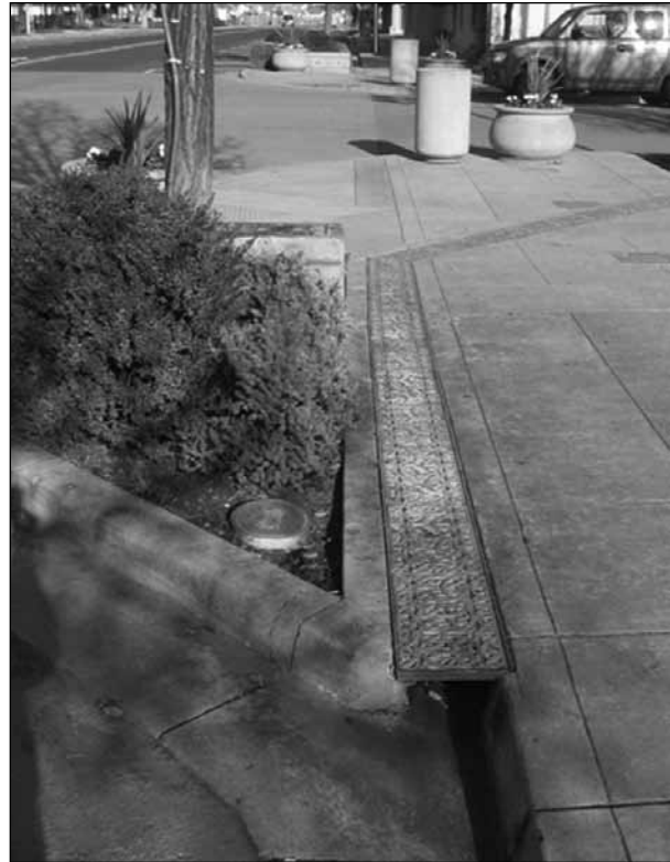
Figure 10.19 Curb extensions may be used as landscaping or hardscape opportunities. This example shows a retrofit curb extension with drainage retained between the extension and the curb. Source: Community, Design + Architecture.
