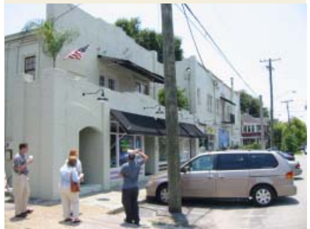
Marybuilt building recent facade improvements: new awnings, coordinated paint scheme, decorative lighting, and restored storefront windows
