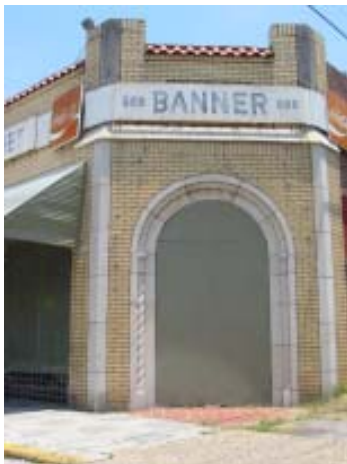
Existing Town Center commercial building that would benefit from facade improvements
