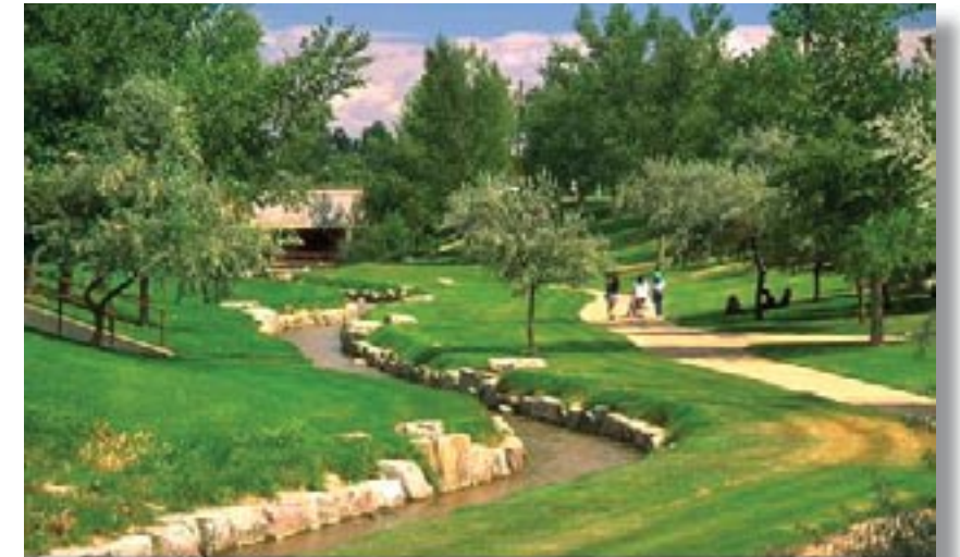
Storm water systems that are part of the natural landscape
