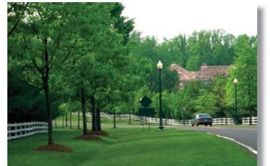
Swales along the road manage storm water while preserving rural character
