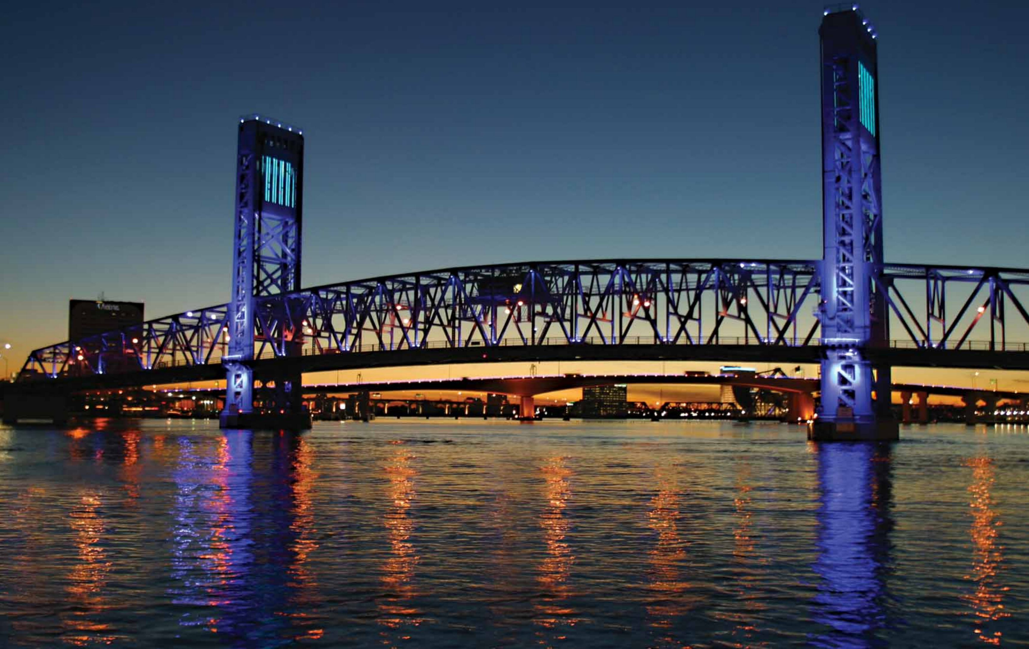
Main Street Bridge
