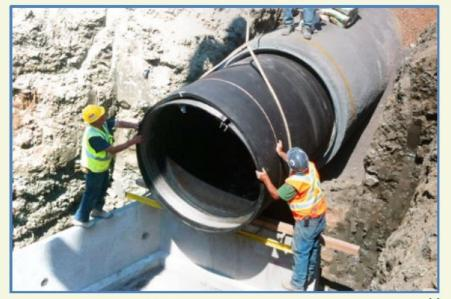
One type of tide check valve, Tideflex CheckMate Inline Check Valve<sup>[6]</sup> will allow stormwater to drain out under lower tide conditions. During high tide, the valve will prevent sea water from backing up into the stormwater pipe network.
