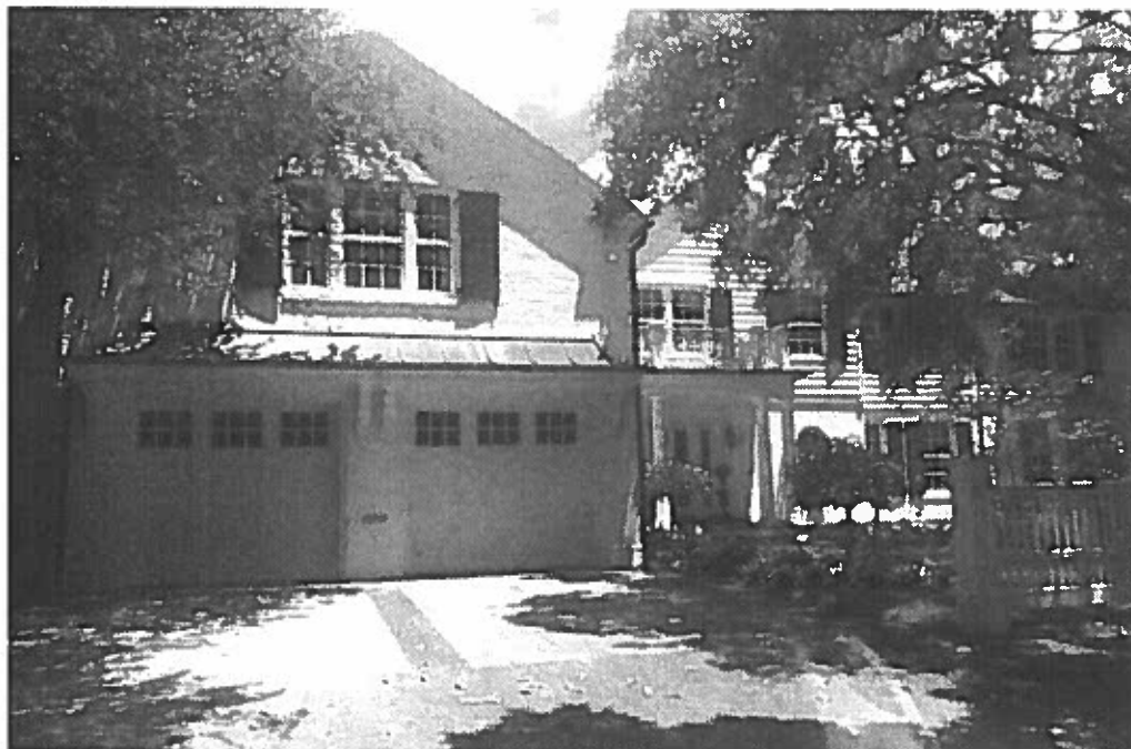
View of Properties to the West (AD-01-36)
