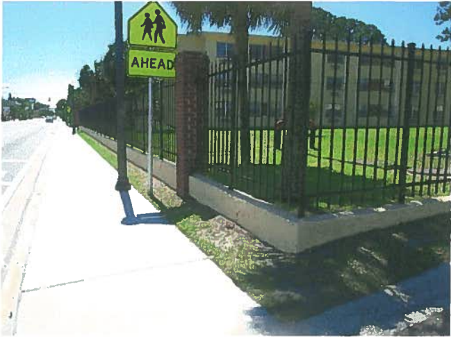
The rot iron fencing is severely rusted and decayed at the bottom and poses a hazard to pedestrians walking by.
