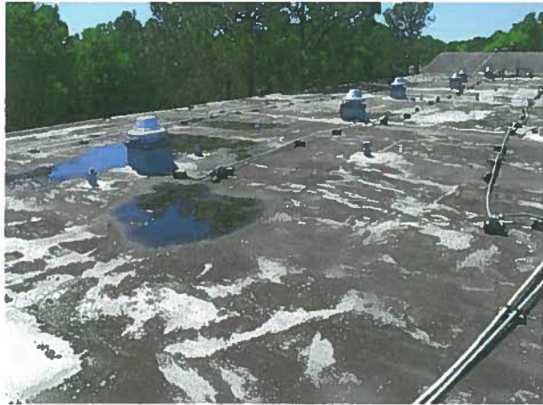
Standing water in certain parts of the roof. Air condition units on blocks and not on proper stands.
