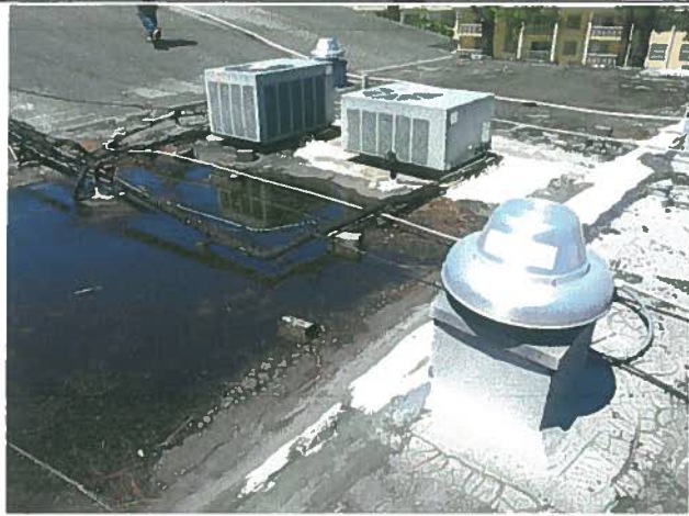
Standing water in certain parts of the roof. Air condition units on blocks and not on proper stands.
