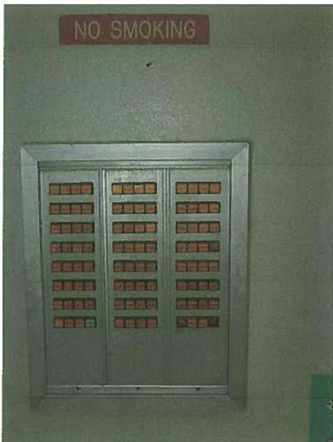
The call center panel is the original system and is obsolete, inoperable and needs to be replaced.
