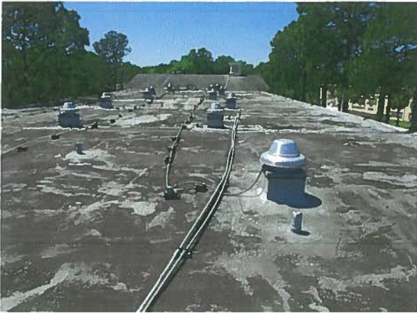
Soft spots and patches located throughout the roof. Some leaks have been reported by residents.
