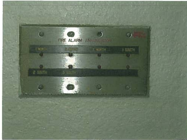
The Annunciator for the fire alarm is obsolete, and needs to be replaced.
