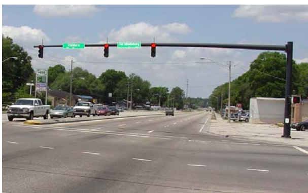
Single mast arm traffic signal at the Old Middleburg Road North intersection
