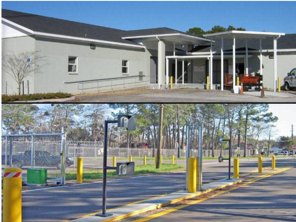
Top: MCC Warehouse Expansion; Bottom: MCC Access Control
