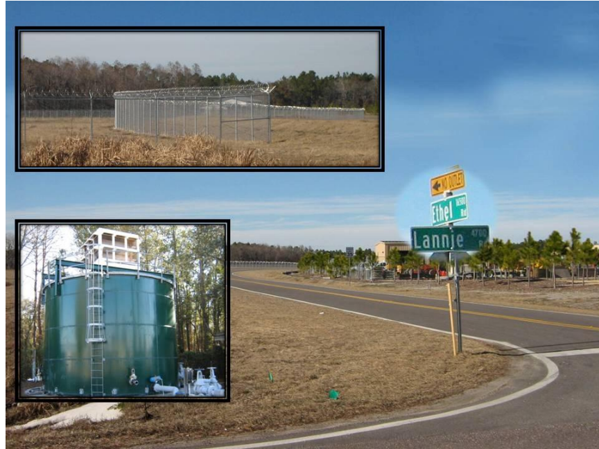
Top Insert: MCC Perimeter Fencing; Bottom Insert: MCC Water Processing Plant; Picture: Newly Rerouted Ethel Road
