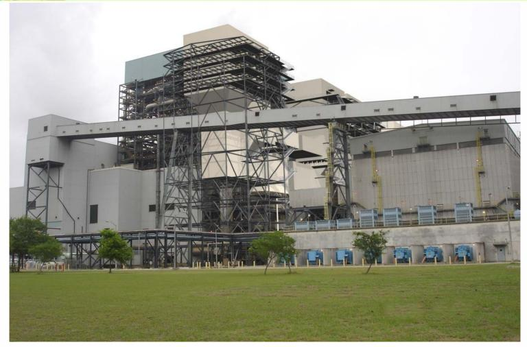
**NEW DUCTWORK WITH REACTOR INSTALLED – WEST VIEW**
