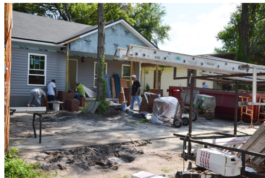
One of the 25 Homes Being Built in One Week by HabiJax
