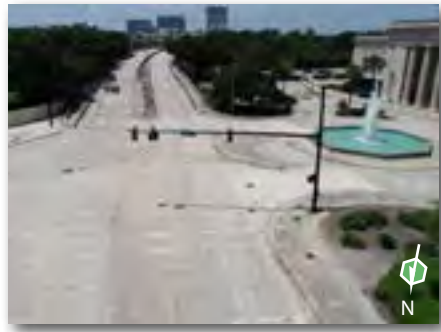
Existing conditions on the Park Street Viaduct
