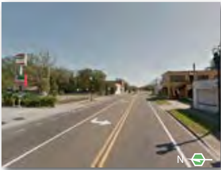
Existing conditions on 8th Street looking east
