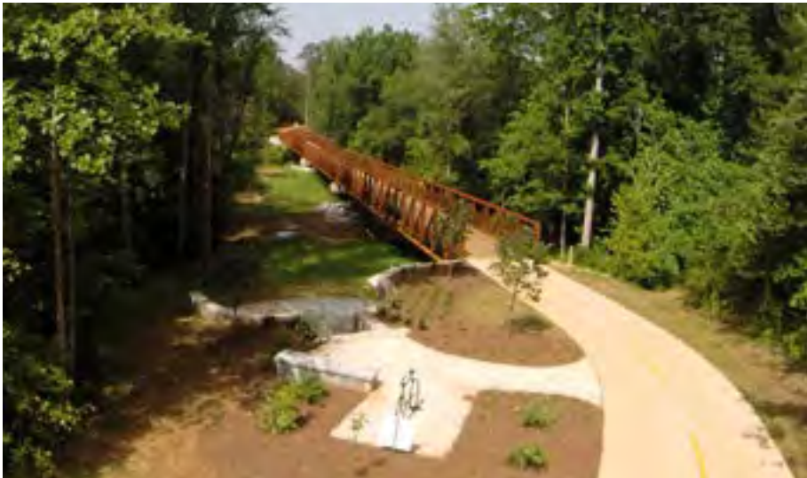
Prefabricated steel bridge allows the trail to cross above existing roads and waterways.
