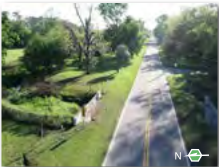
Existing conditions on McCoys Creek Boulevard looking east
