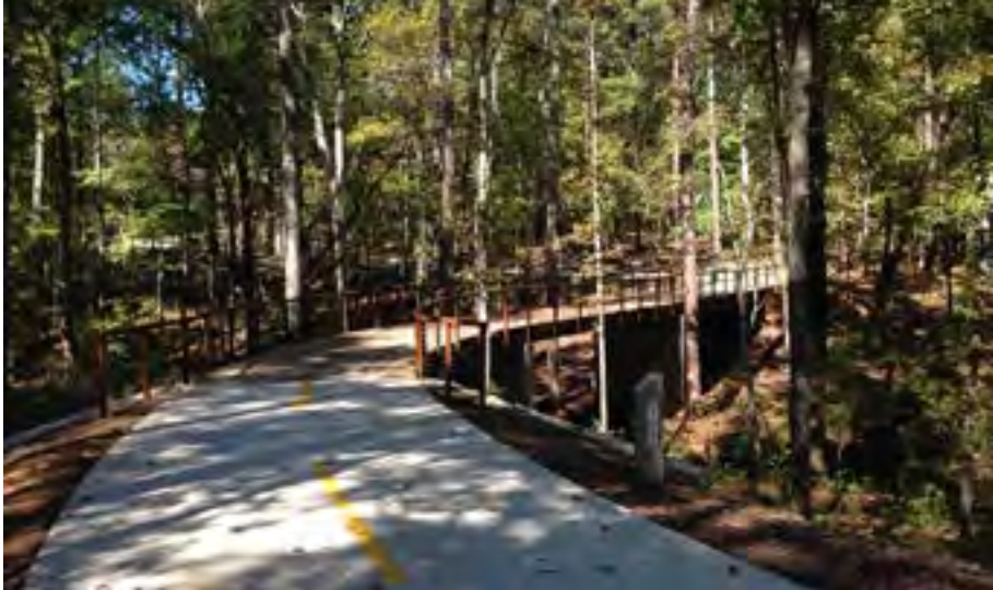
Custom steel bridge allows the trail to naturally blend into wooded areas.
