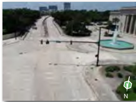
Existing conditions on the Park Street Viaduct
