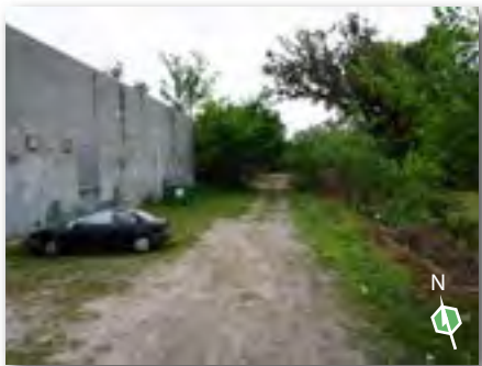
Existing conditions on the abandoned rail corridor
