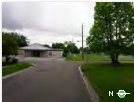
Existing conditions on Placeda Street looking east towards Line Street
