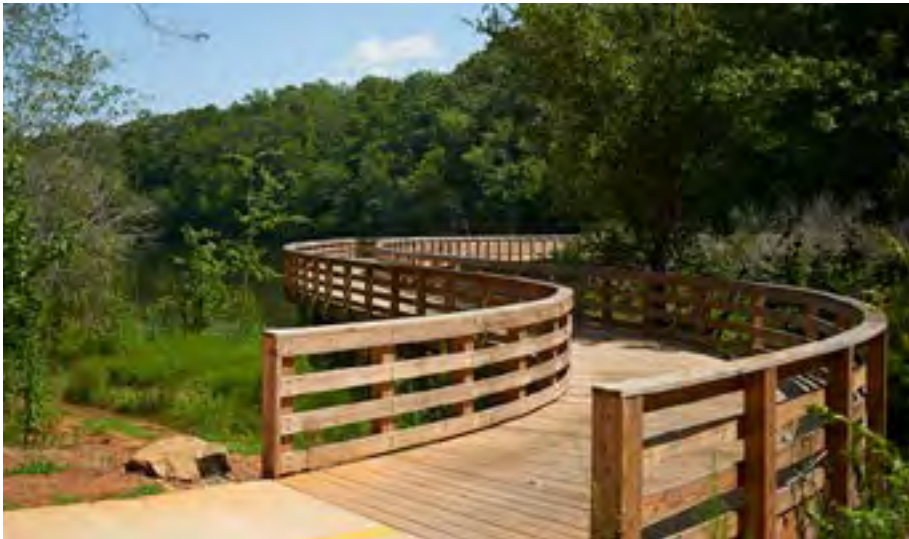
Wooden boardwalk structure for crossing lakes and wetlands.
