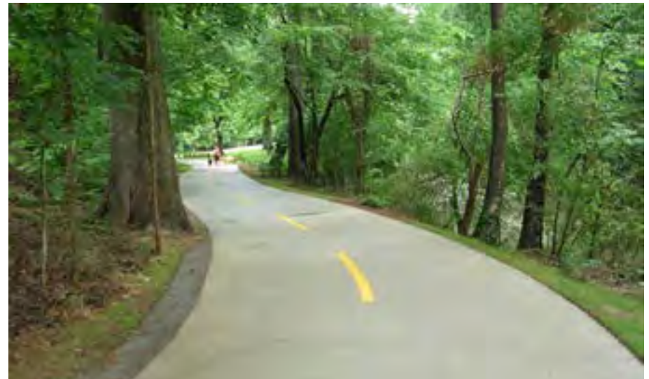
An example of incorporating the pervious concrete strip along the trail edge
