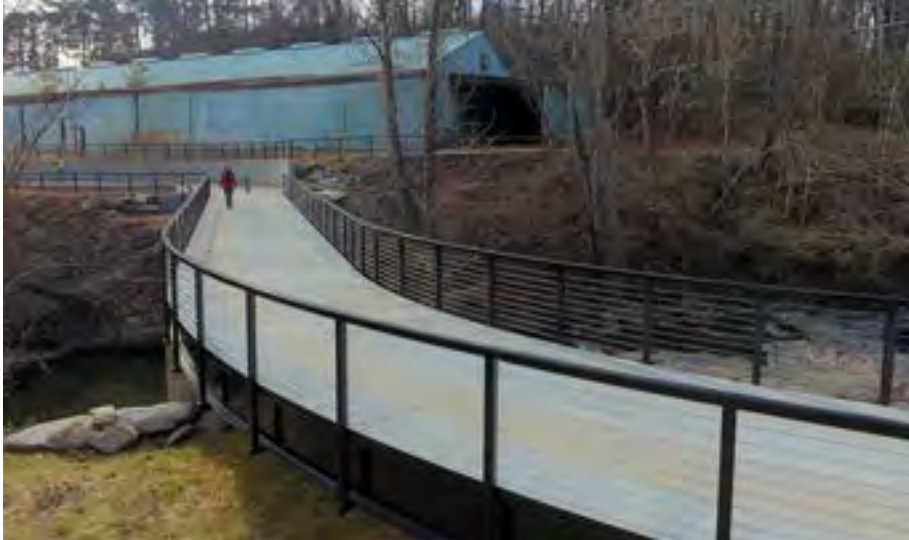
Bridges with painted finishes are timeless and suitable for urban environments
